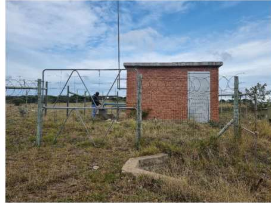
Domestic Water Supply Production Boreholes in Port Alfred (Borehole ID: P4N0011 )
