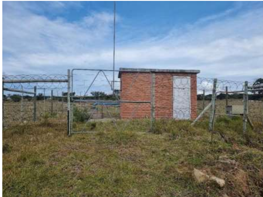
Domestic Water Supply Production Boreholes in Port Alfred (Borehole ID: P4N0012)
