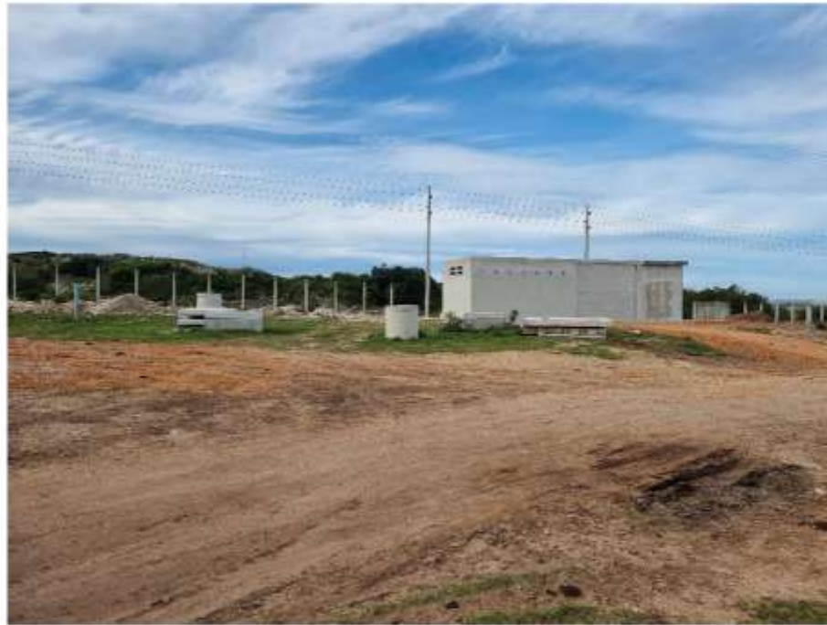
Production Borehole within the Coega Ventershoek Wellfield
