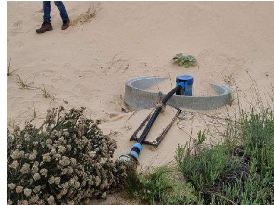
Production Borehole in the Boesmansrivier Wellfield in Port Alfred
